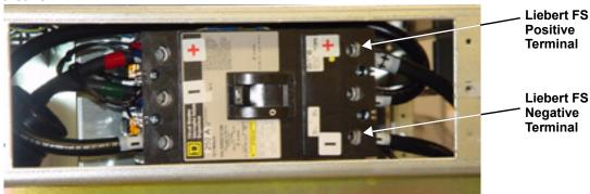
The Liebert FS cabinet is configured for top entry cables in standard configuration. The cables can also be run through the side panels. The Liebert FS cabinet does not accommodate bottom entry cables.
